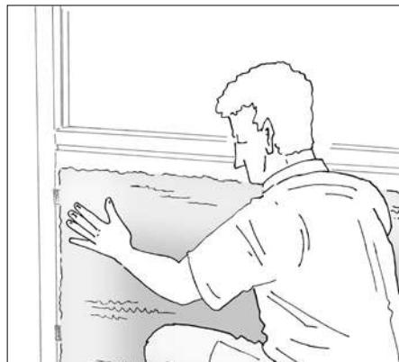
► Fill the cavity with insulation in accordance with specification (insulation not supplied by VELFAC). NB. Vapour barrier is integrated with backboard.
